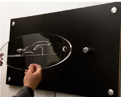
In this example, the backer panel is mounted using a standard low profile cap and barrel in the drywall.
